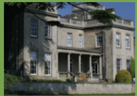
6. Brackenhurst Hall, the focal point of the campus
