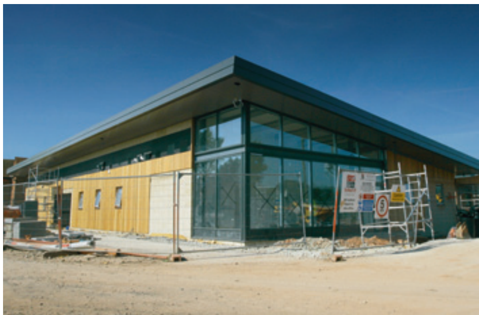
Work on the new veterinary nursing building is now underway
